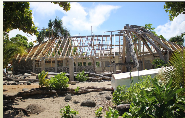
Good building structure using local materials in Emau Island.
